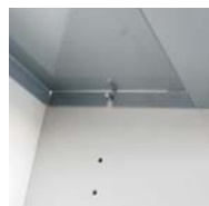
Precautionary fixing of metal shelves
