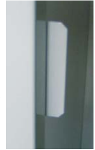
2 Lock reinforcement (surcharge)
